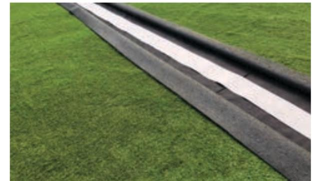
Unroll the Luxigraze Jointing Tape, green (shiny) side down, along the entire length of the join. Secure in place, to stop the tape moving.
